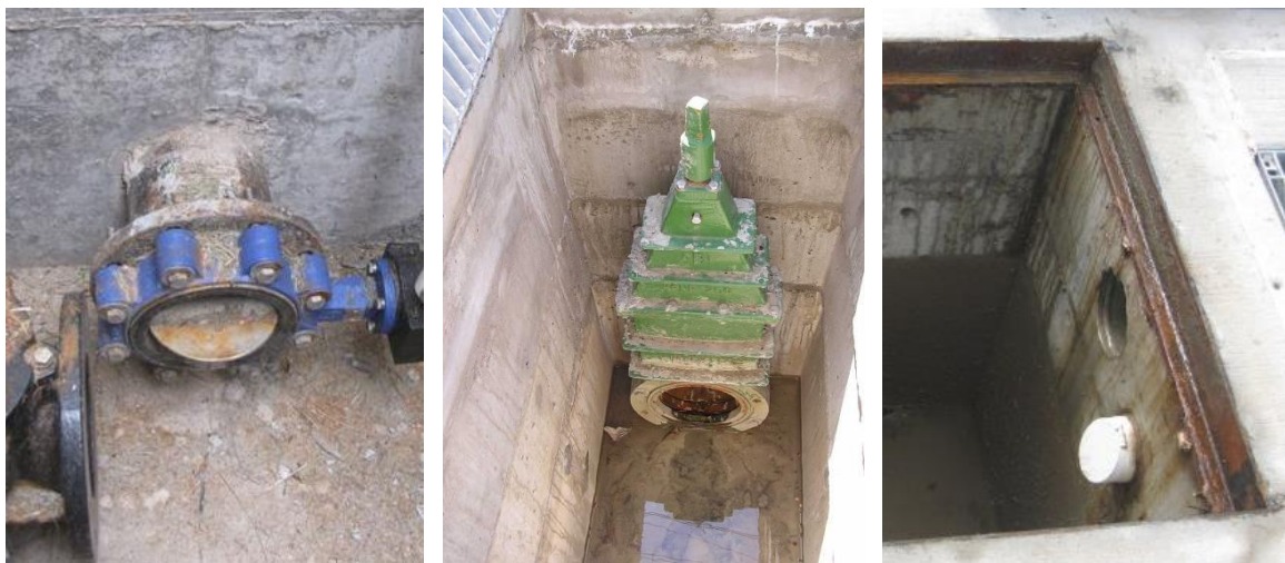
Figure 9: Butterfly, Knife Gate and Reflux Valves (left to right)
