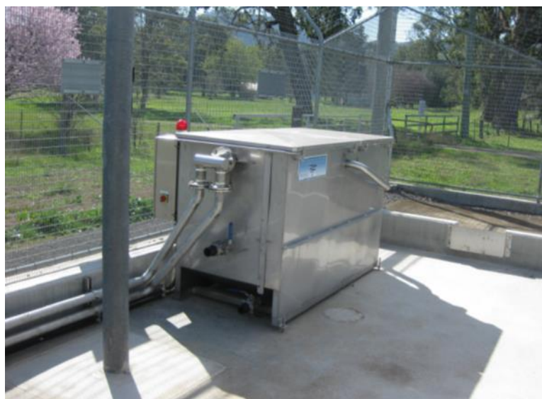
Figure 10: Typical Parallel Plate Separator
