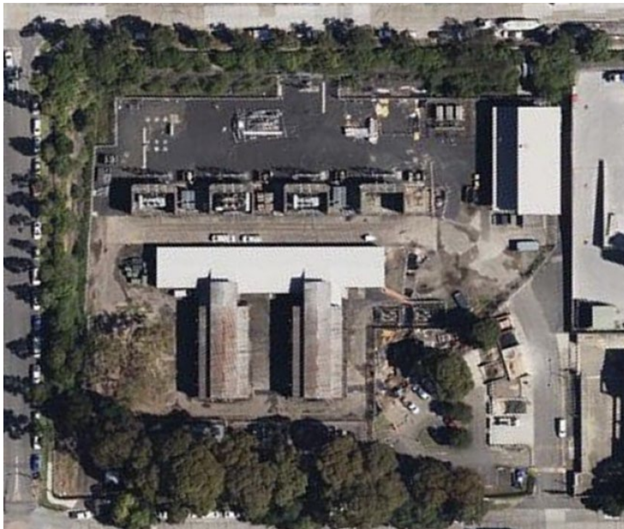
Figure 2.2 – Willoughby STS aerial view
