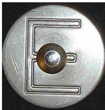
Figure 13: Approved kerb marking
