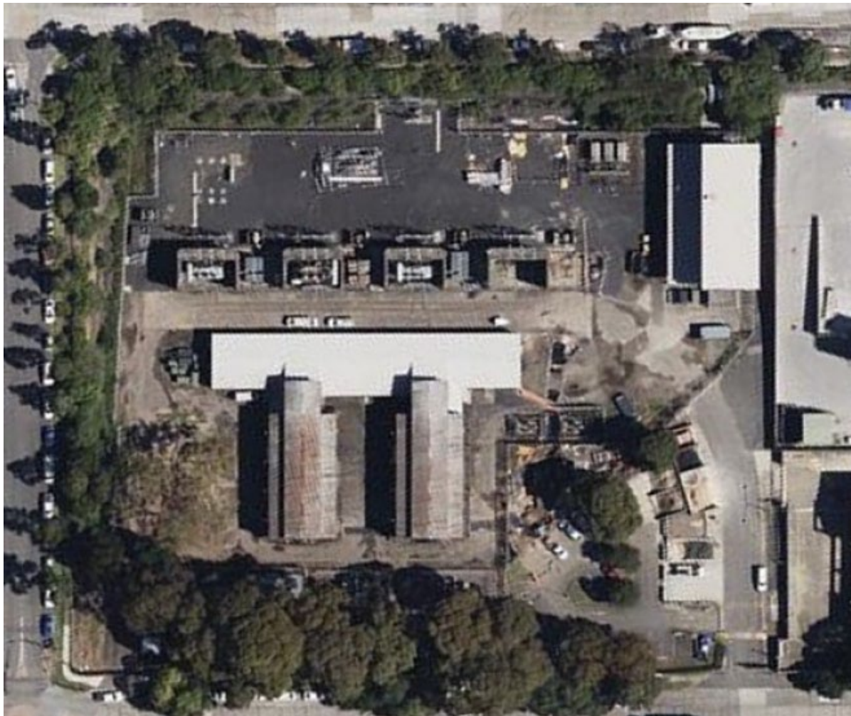
Figure 2.2 - Willoughby STS aerial view
