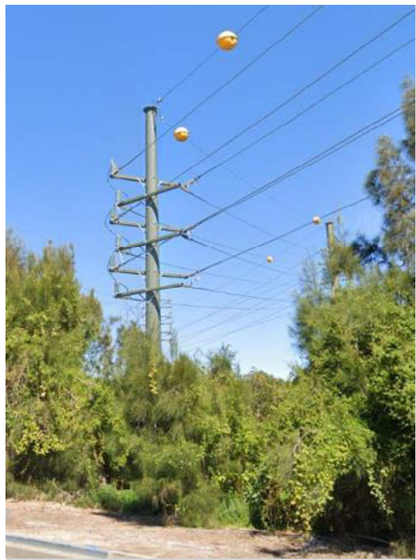
Marker balls near an urban helipad
