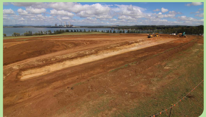
Construction at the new Antiene substation, Muswellbrook
