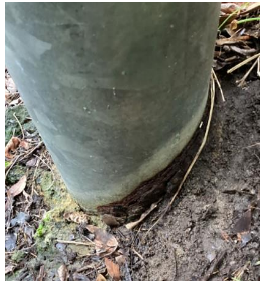
(h) Defect notice
