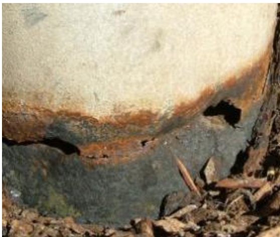
(k) Emergency Line and Defect notice
