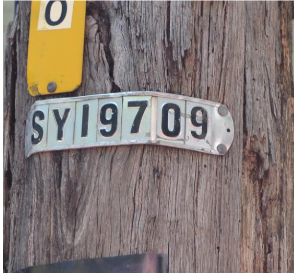
Figure 8.2 - Example of a slide-in character label on a timber pole
