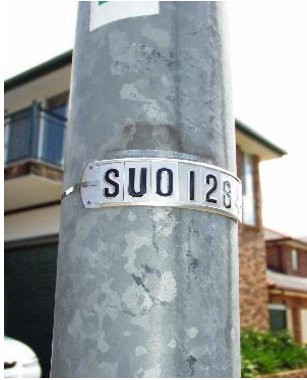
Figure 8.3 - Identification label on steel street lighting column
