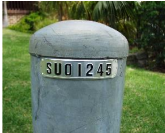
Figure 8.10 - Steel round cover pillar
