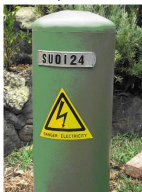
Figure 8.8 - Polyethylene plastic round cover pillar
