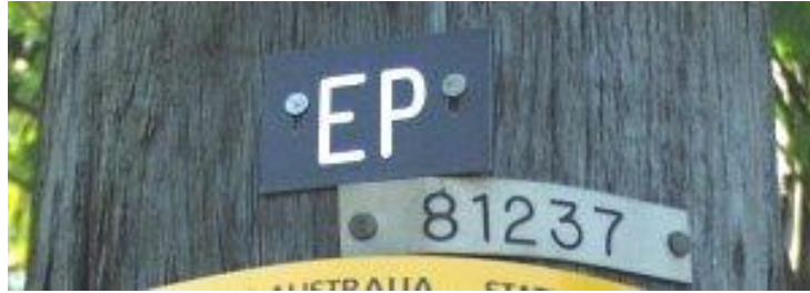
Figure 5.2 - Two labels used to identify a pole
