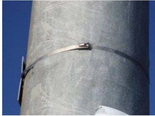
Figure 8.4 - Trim excess length cable tie flush with joiner
