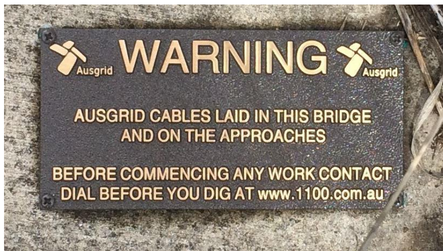
Figure 3 - Example of warning sign for bridge installation
