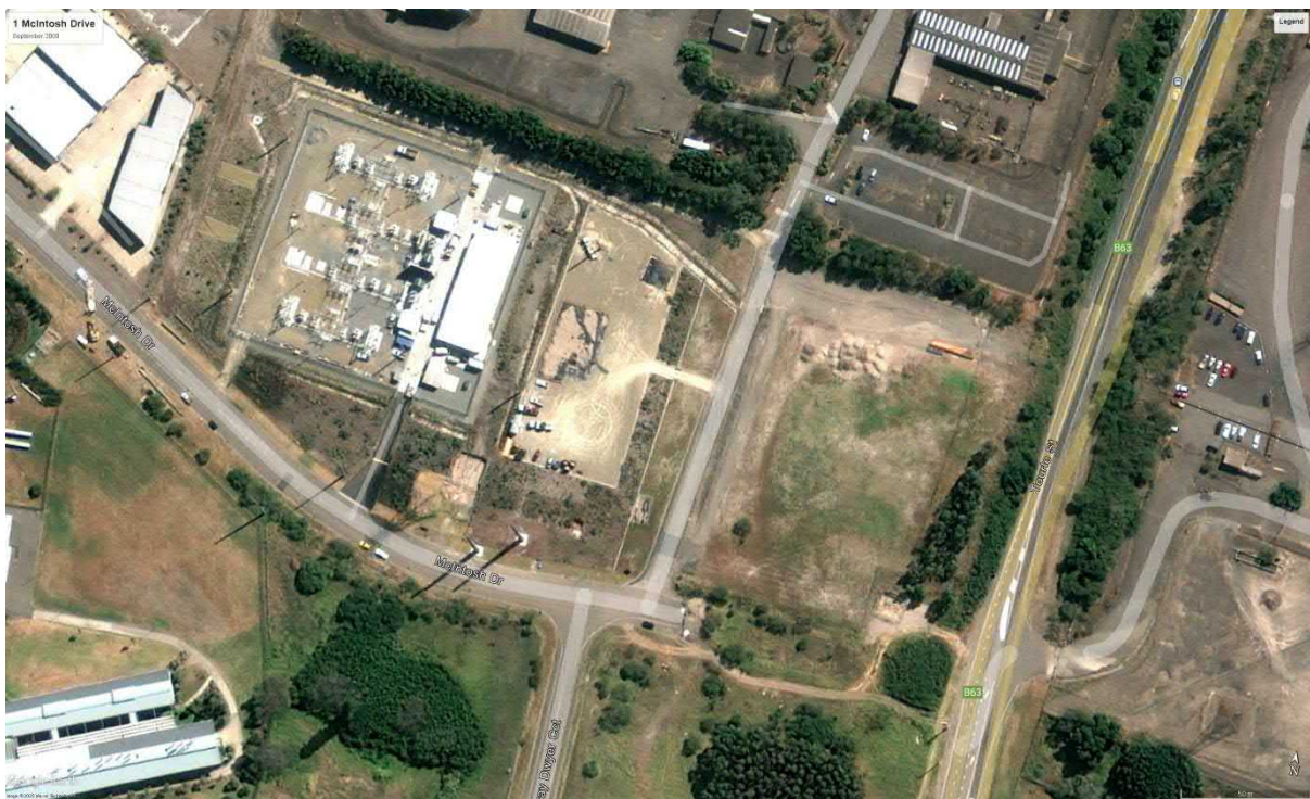
Plate 3.1: Aerial imagery of 1 McIntosh Drive before planting (September 2009)
