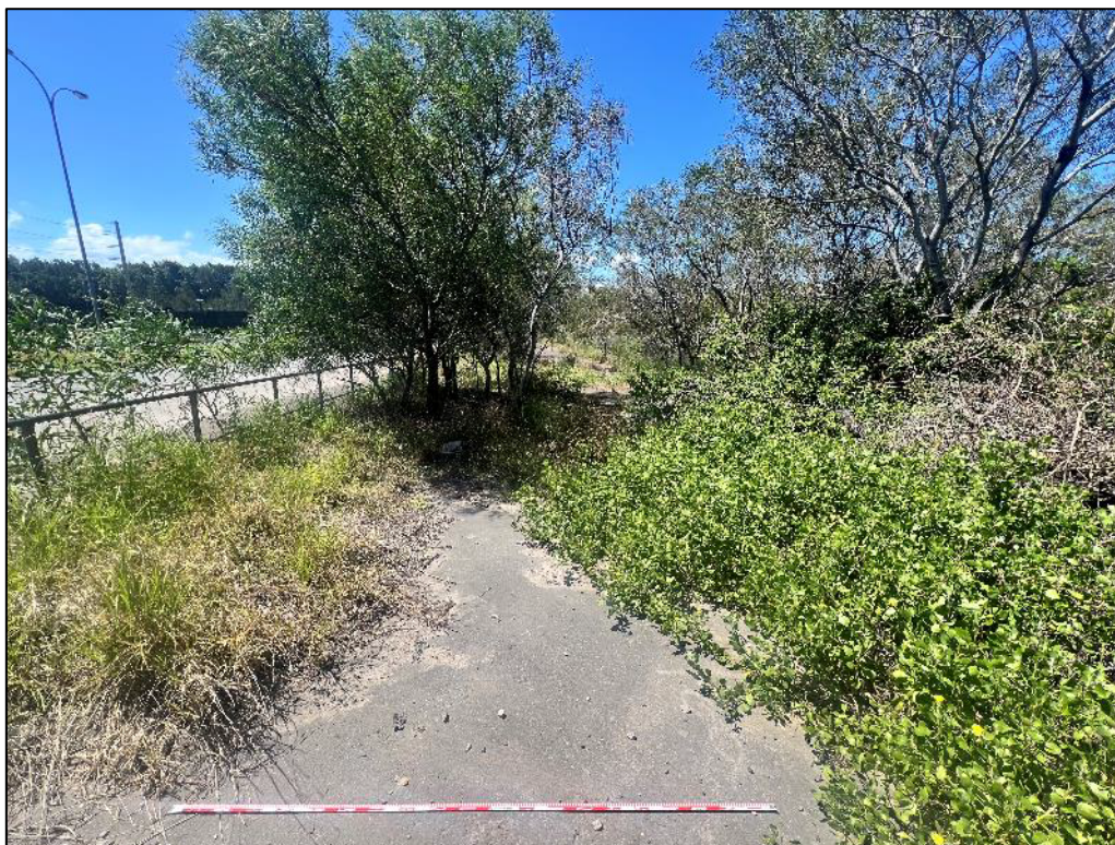
Plate 2: Looking north along existing bitumen hardstand within eastern portion of the study area.
