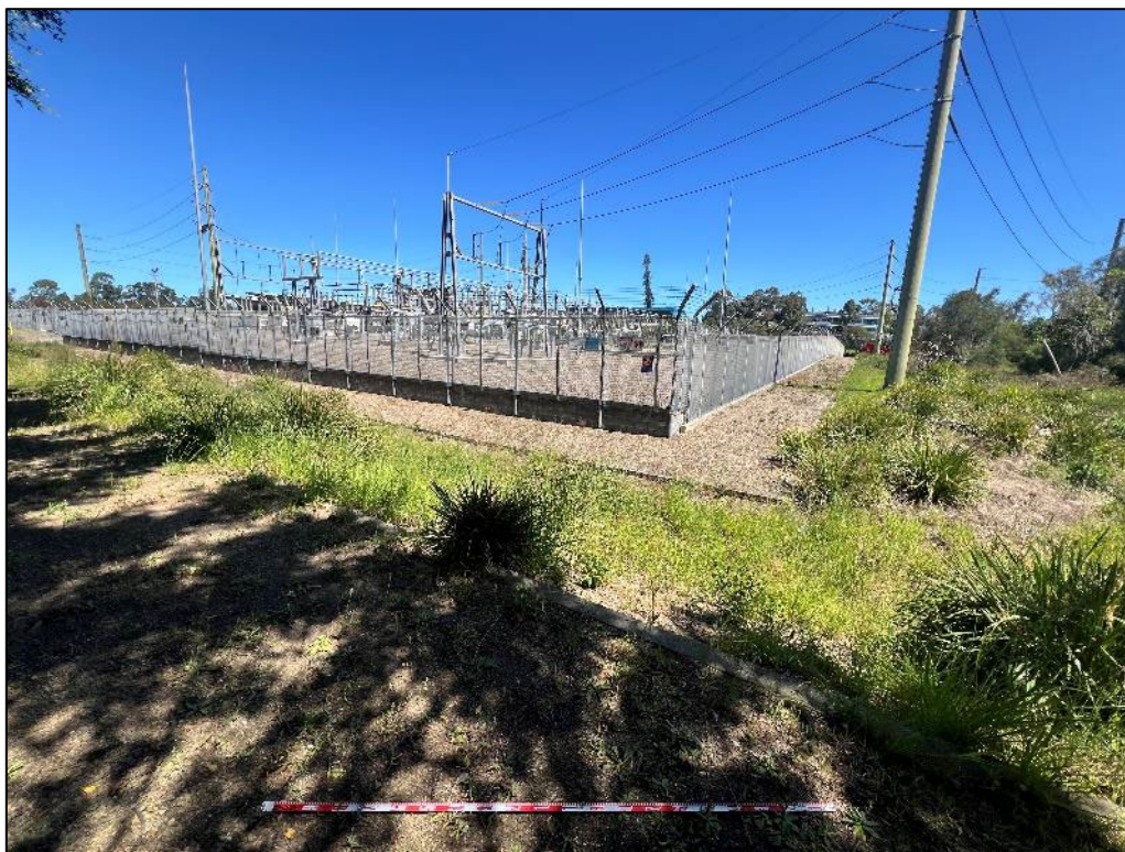
Plate 10: Looking south east across the site.
