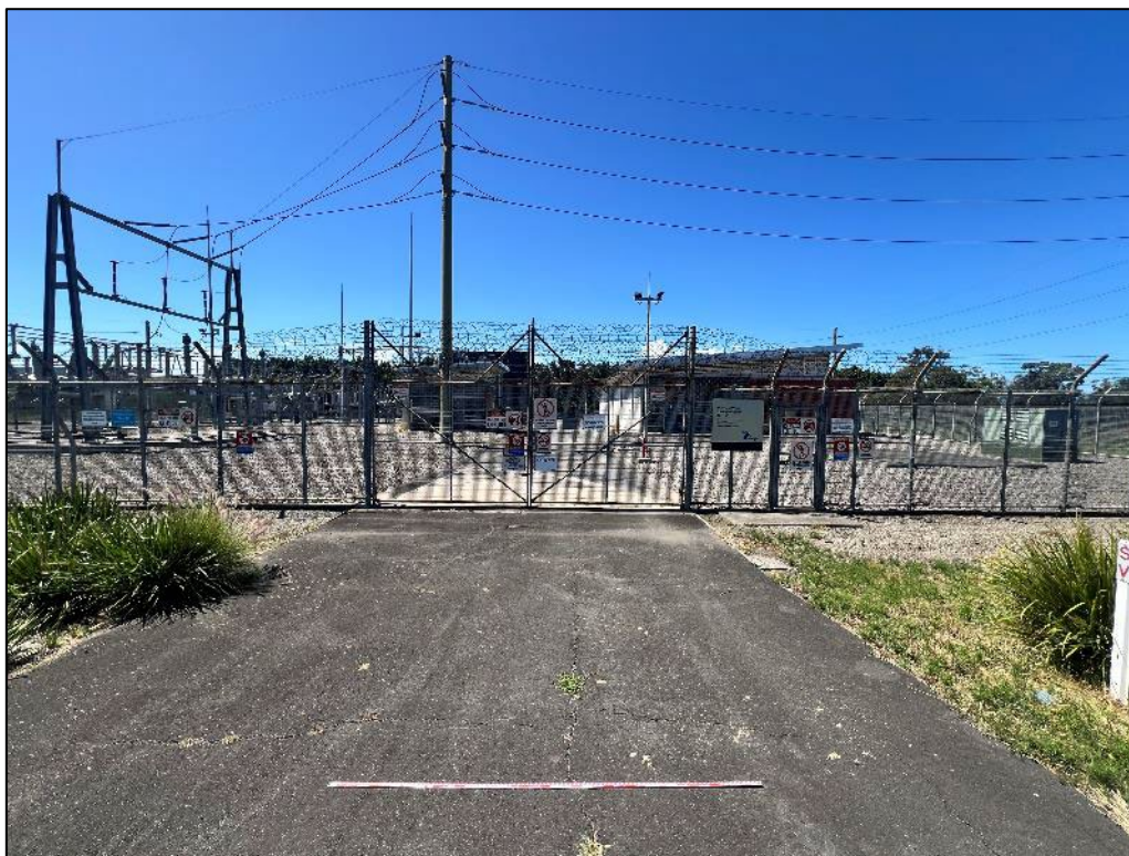
Plate 6: Looking north in to the frontage of the existing Zone Substation.
