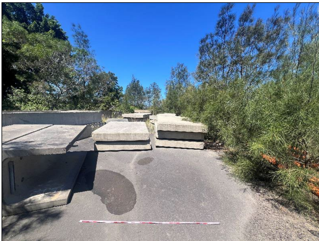
Plate 4: Concrete casing for underground services stored within the northern portion of the site.
