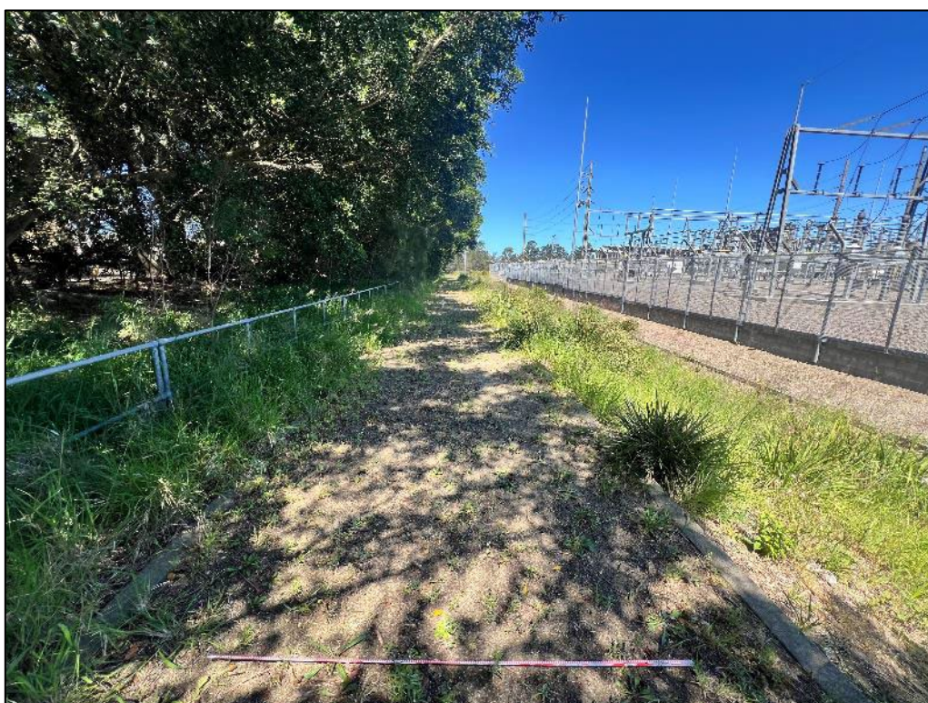
Plate 9: Looking east along the northern boundary directly behind the Zone Substation.
