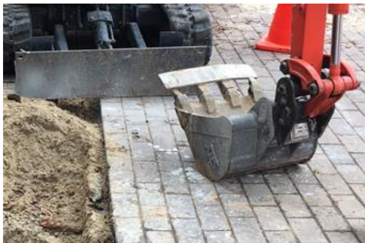
Figure 2: Example of excavator bucket without exposed teeth.
