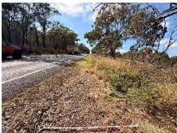
Plate 14: Looking east along Mitchell Line of Road along HCC REZ alignment deviation.
