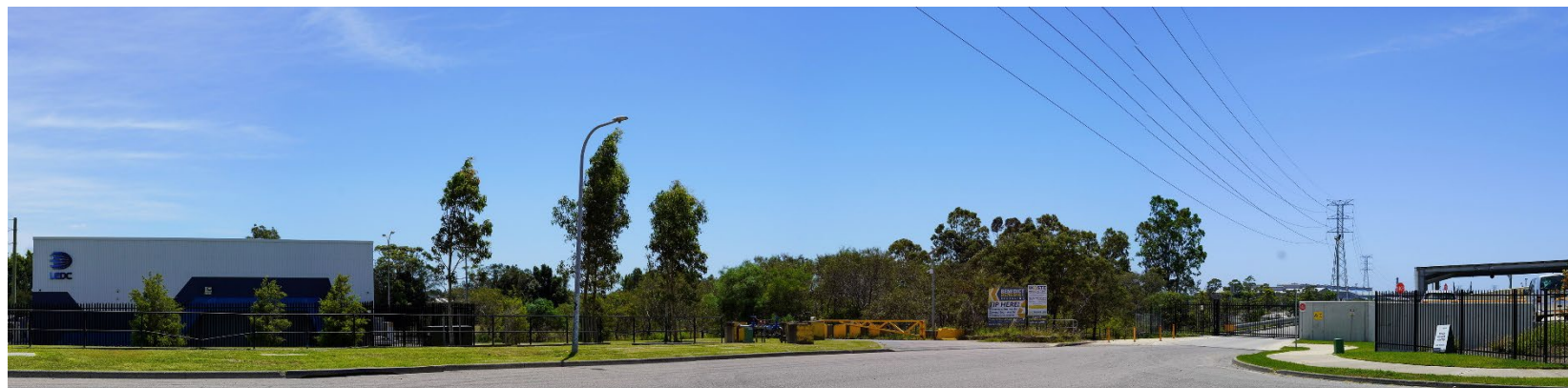
Figure 6-2 VP1: McIntosh Drive looking east towards the Project
