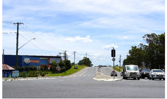
Figure 5-8 Views looking north towards the site from Tourle Street / Industrial Drive
