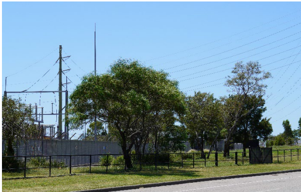
Figure 5-3 Views looking east towards the site from McIntosh Drive
