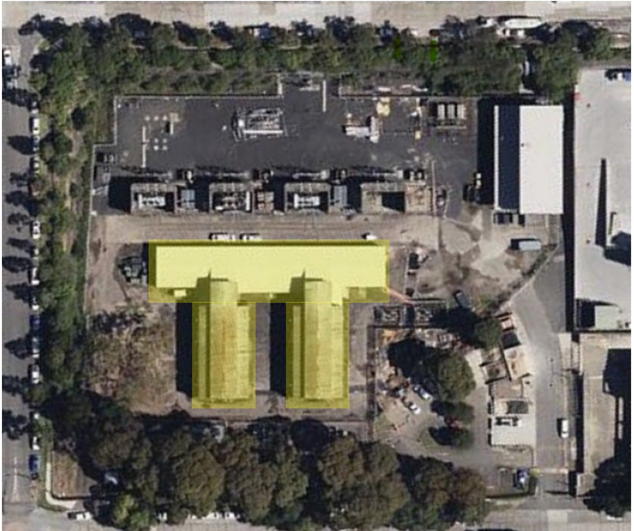
Figure 2.2 – Willoughby STS aerial view
