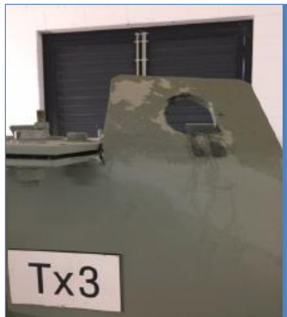
Figure 2: Distorted 10mm thick lifting lug, and damaged tank lid weld.
