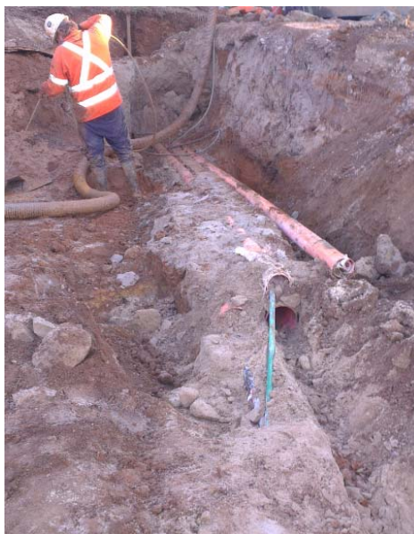
Picture: trench with conduits encased with stabilised sand
