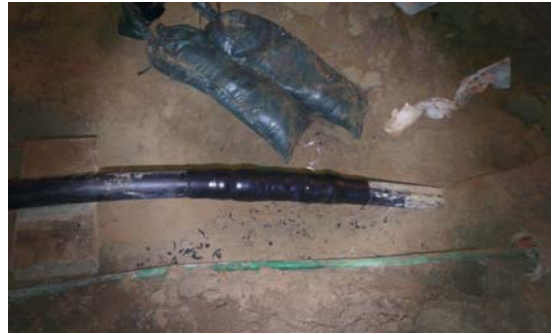
Picture: repaired 33kV underground cable
