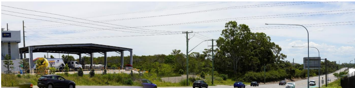
Figure 6.4-6: VP3 Tourle Street, looking northwest towards the Project (Aurecon, 2025)
