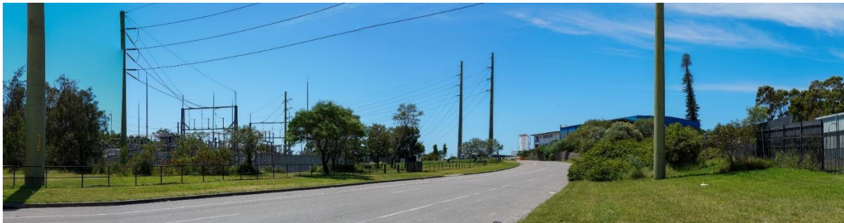
Figure 6.4-5: VP2 McIntosh Drive, looking northeast towards the Project (Aurecon, 2025)
