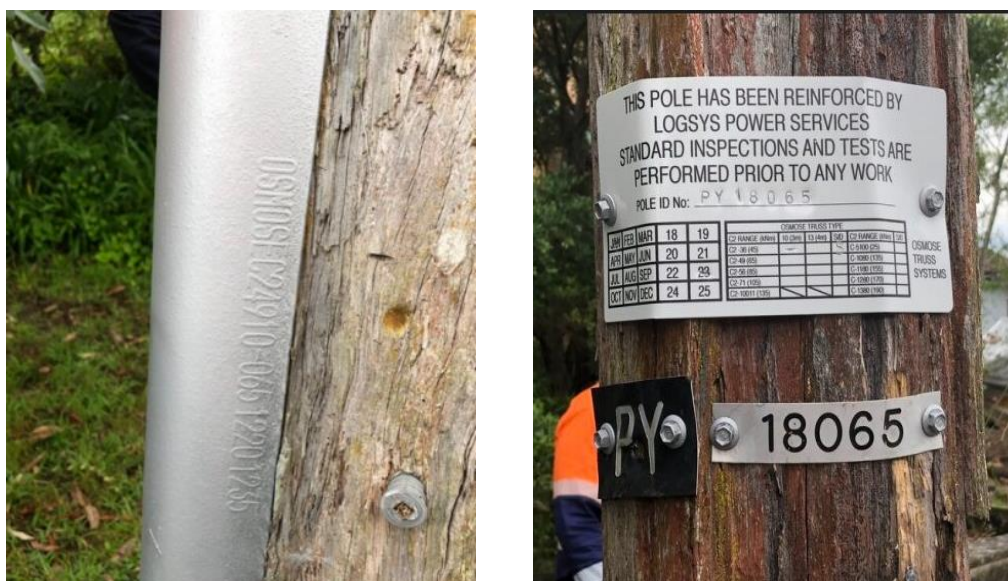
Figure 10 – Examples of Osmose Osmo-C-Truss embossed details and pole label
