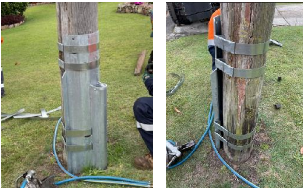
Figure 13 – Powerbeam nail secured with bands
