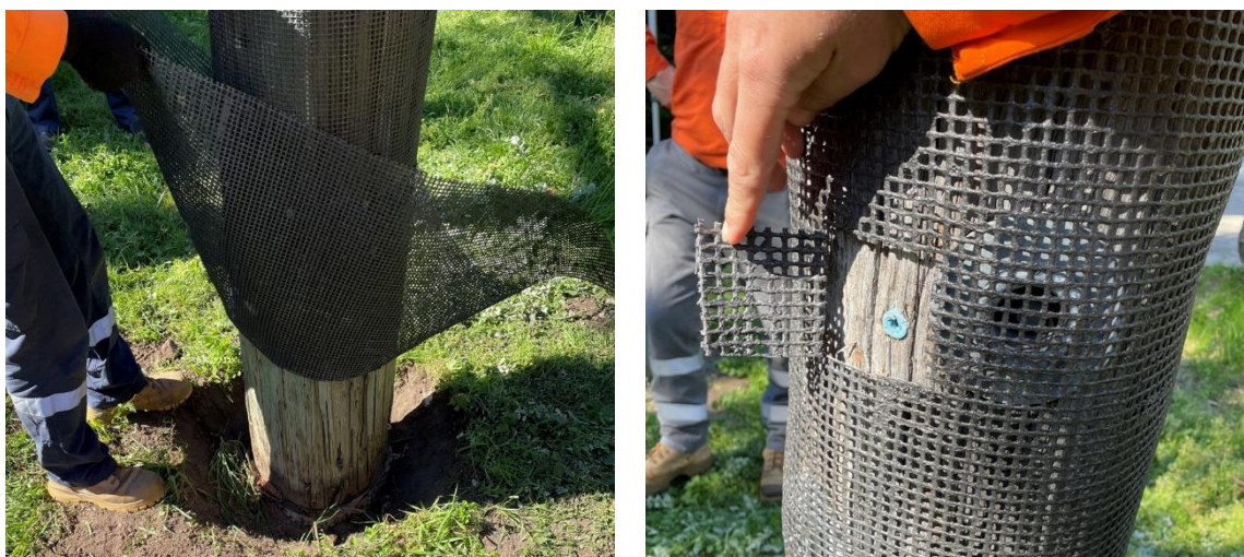
Figure 16 – Examples of partially removing or cutting Genics fire mesh for pole inspection
