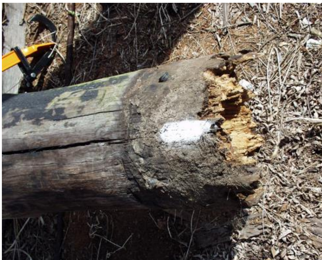
Figure 35 – Damage Caused by Glyptotermes At and Below Groundline
