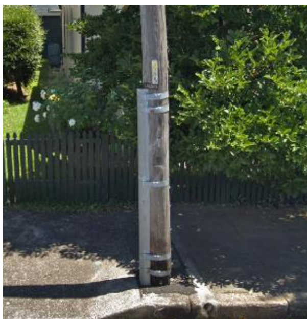
The Osmose (Logsys) 'Osmo-C-Truss' or 'Osmo-C2-Truss' splints are of similar appearance and design to Ausmose Oz C splints however, the splints are embossed vertically along the above ground length of the splint with the splint details and a label for the splint details is attached to the pole above the splint (refer to Figure 10). Osmo-C-Truss splints are typically used for poles with a large diameter and Osmo-C2-Truss splints are used for typical distribution poles due to their lighter weight design.
