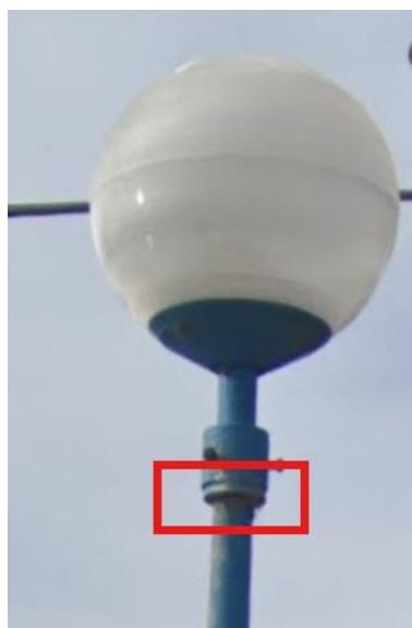
Figure 18 – Examples of insulating spigot installations
