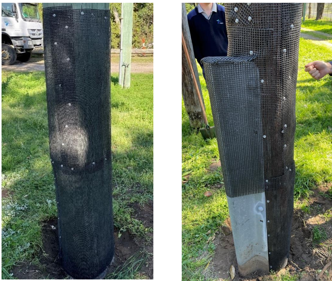
Figure 15 – Examples of Genics fire mesh installed on timber poles
