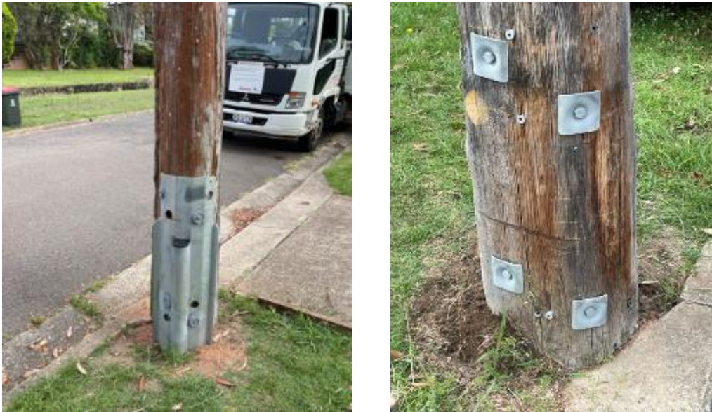
Figure 12 – Powerbeam nail secured with bolts
