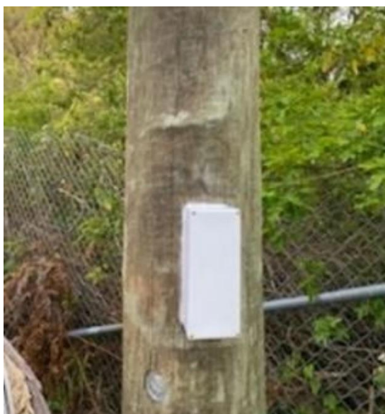
Figure 49 – Installed Termatrix Bait
