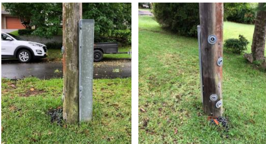
Figure 11 – RFD nail secured with bolts
