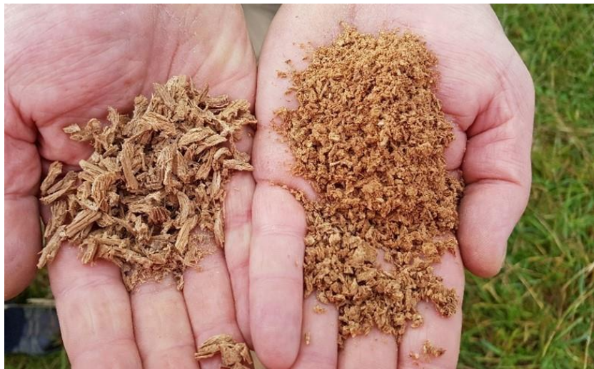
Figure 47 – Example of large shavings from good timber (left) compared to small shavings from decayed timber (right) from the same pole
