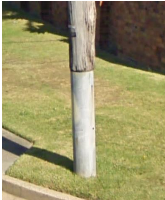
Figure 14 – Example of a composite timber pole
