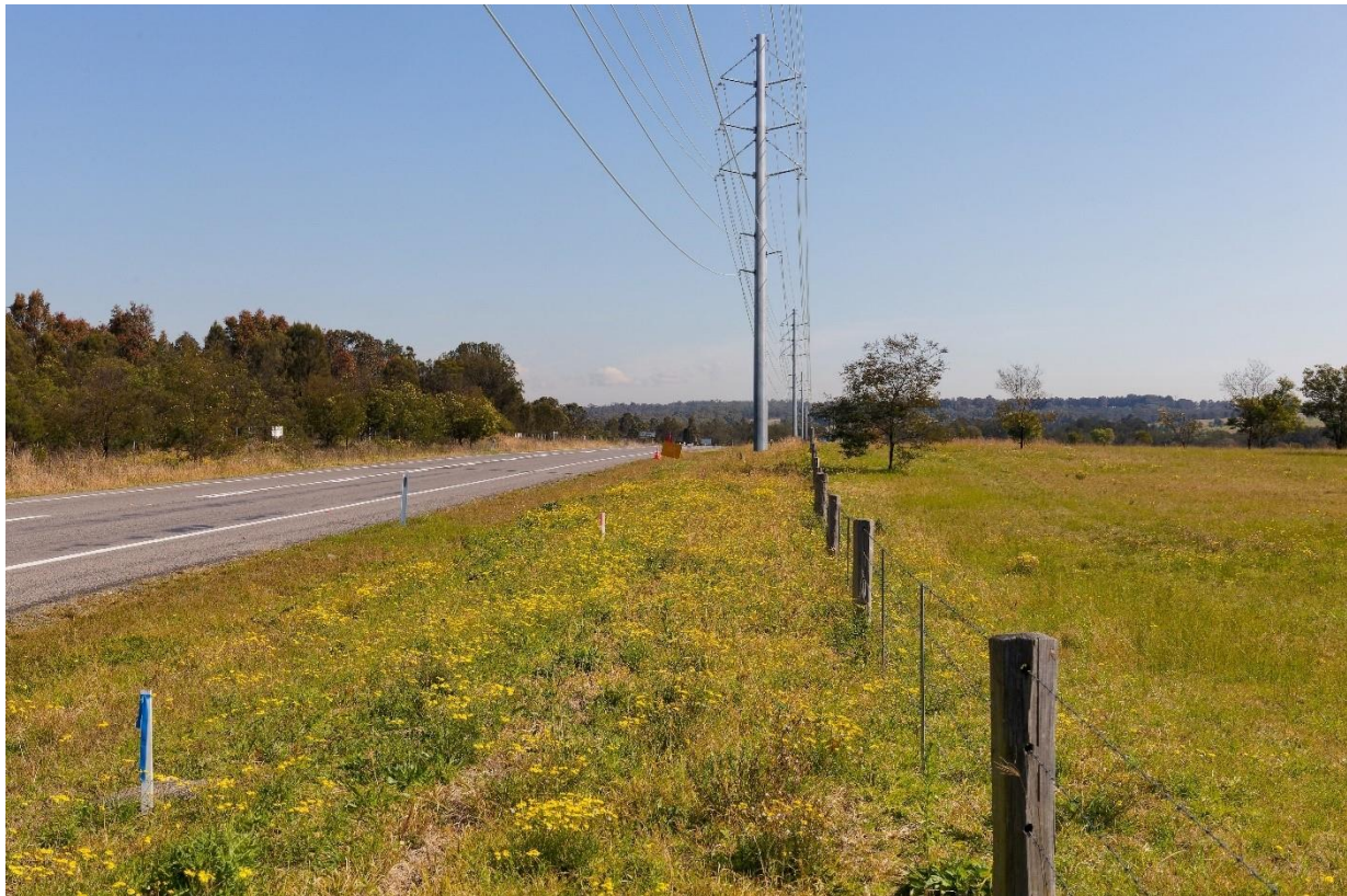
Figure 6-2 Photomontage of a typical powerline and power pole (Source: Ausgrid, 2025)
