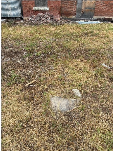
Figure 4-19 Extant foundations for outbuildings (Source: AECOM 2025)
