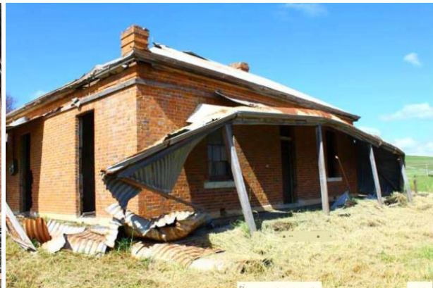
Figure 4-8 2015 Northern elevation comparison (Source: CMP, 2015)
