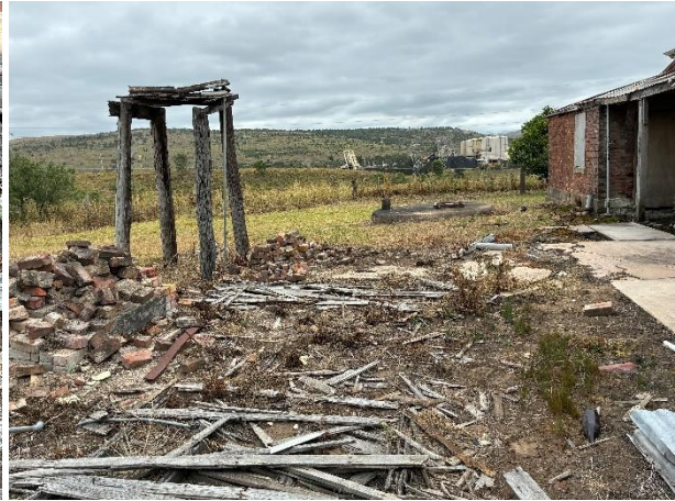
Figure 4-16 Remains of outbuildings (Source: AECOM 2025)
