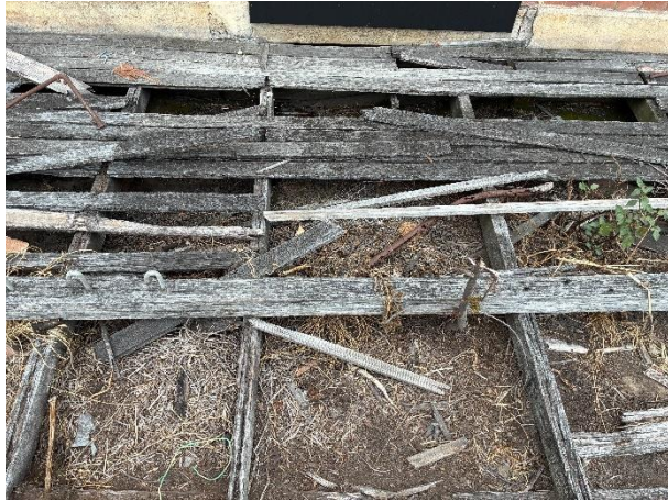
Figure 4-15 Eastern deck (Source: AECOM 2025)
