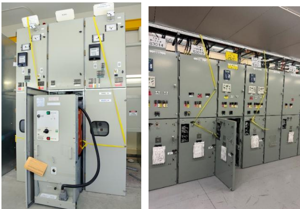
Figure 34 – Examples of barrier-out method used on indoor metal-clad switchgear
