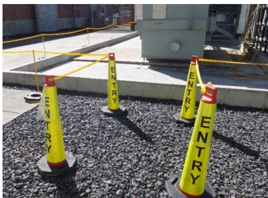
Figure 30 – A photograph and diagram illustrating correct entry to a safe work area with the entrance corridor tape formed at right angles to the safe work area.
