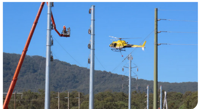
Recent helicopter stringing covering a distance of 4km in Muswellbrook
