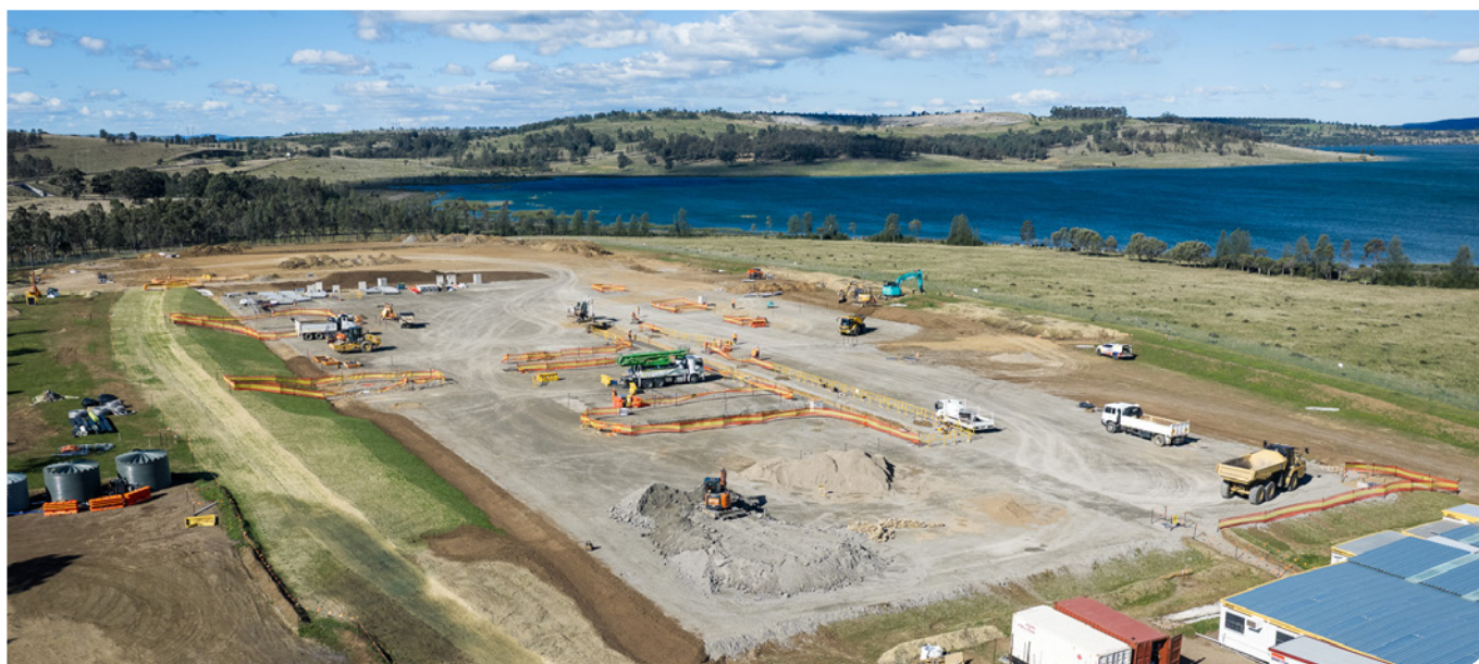
Earthworks progress on site at our Antiene substation in Muswellbrook
