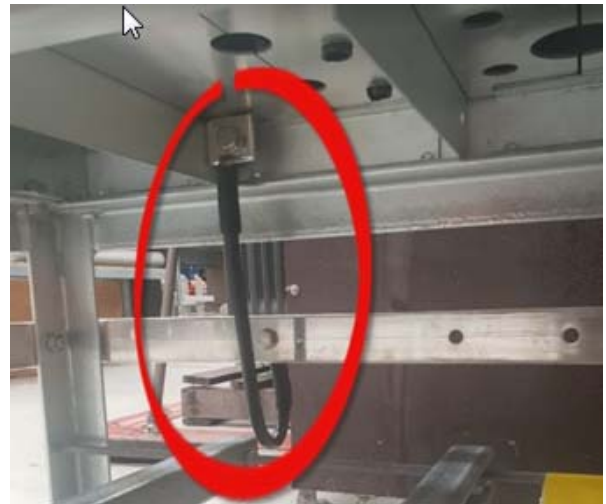
70mm Cu cable (Chamber installation)
