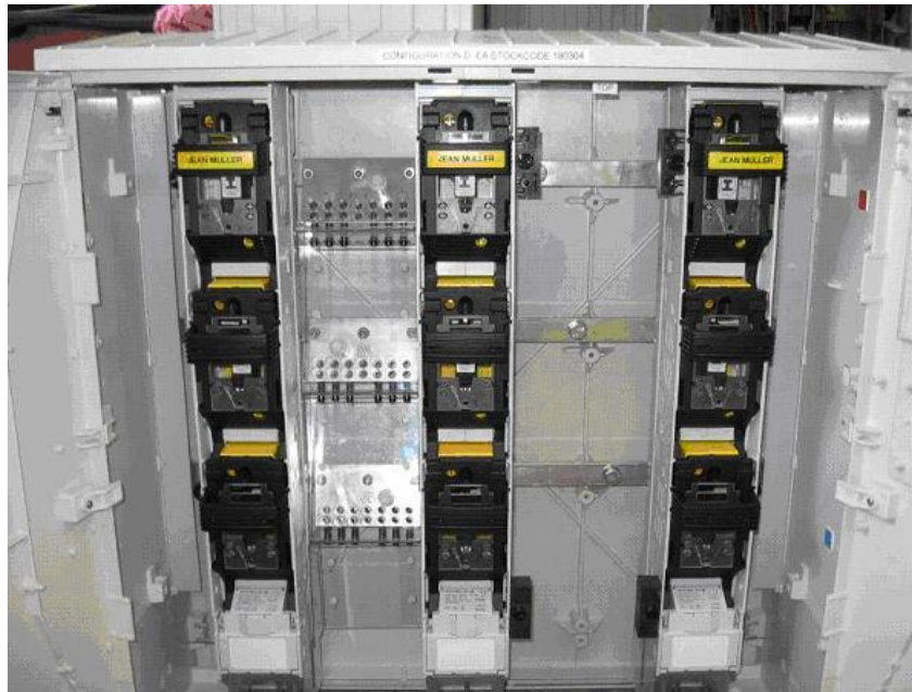
Figure 11 - 3 distributor link arrangement – Configuration D
