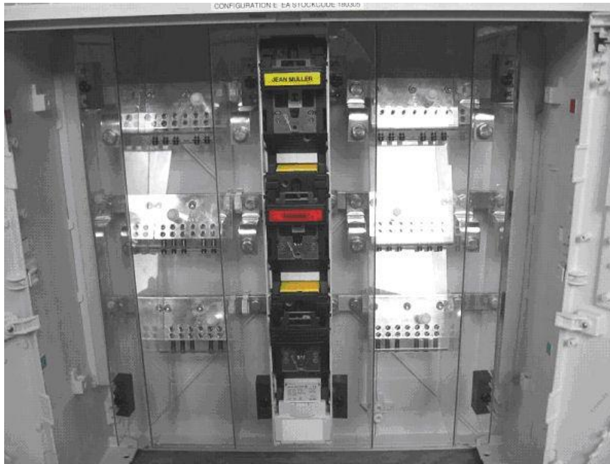
Figure 14 - 2 distributor single link arrangement – Configuration E
