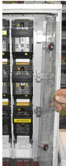
Figure 46 - Polycarbonate cover removed
