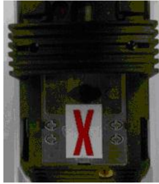
Figure 105 - Cross power source label on link handle
