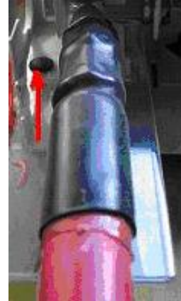
Figure 35 - Phase Barrier viewed from the side of the Distributor Switchgear Module
