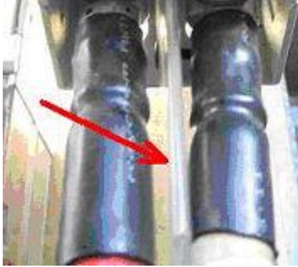
Figure 34 - Phase Barrier viewed from the front of the Distributor Switchgear Module
