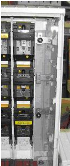
Figure 45 - Polycarbonate cover installed
