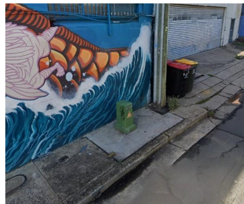
Fig B18 – Unacceptable – Low pillar in line with other assets, but on a narrow footpath. A commercial pillar would be suitable for this location.
