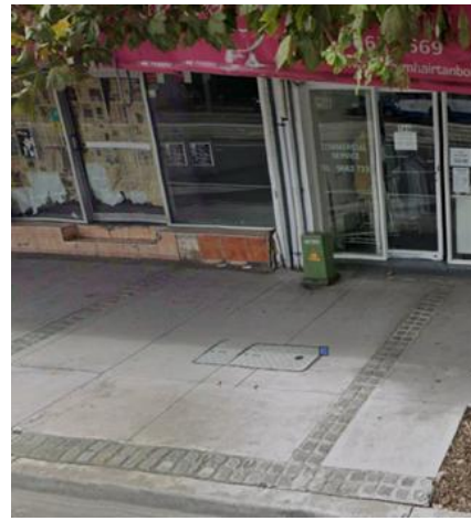
Fig B22 - Unacceptable – Low pillar in a commercial footpath, located in front of a glass panel. A commercial pillar would be suitable using clearances per Table 1.
