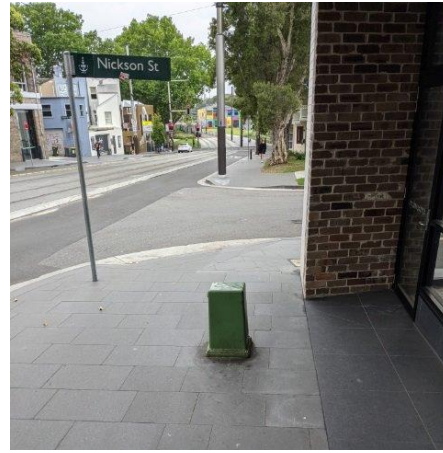
Fig B20 - Unacceptable – Near a doorway and middle of footpath with building line setback.
