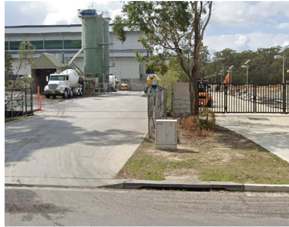
Fig B29 - Unacceptable – Requires additional setback from industrial driveway (LHS) and/or bollards to reduce the risk of large vehicle impacts.
