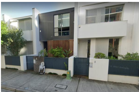
Fig B5 - Unacceptable – Too close to front gate exit. A commercial pillar is also suitable for this area using clearances per Table 1.
