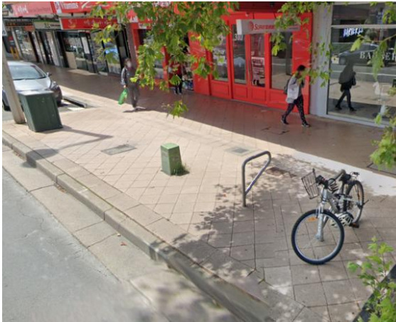
Fig B19 -- Unacceptable – Low pillar in a commercial footpath and more than 1m from other fixed assets. A commercial pillar would be suitable for this location.
