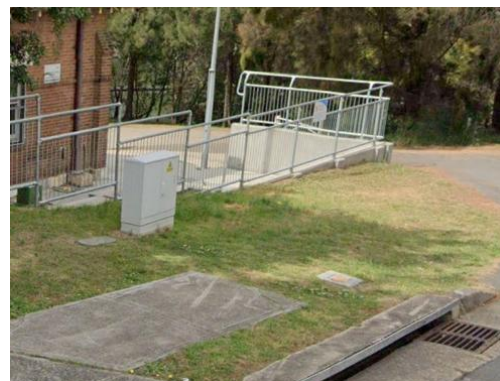
Fig B10 - Good – Clearances per Table 1 maintained.
