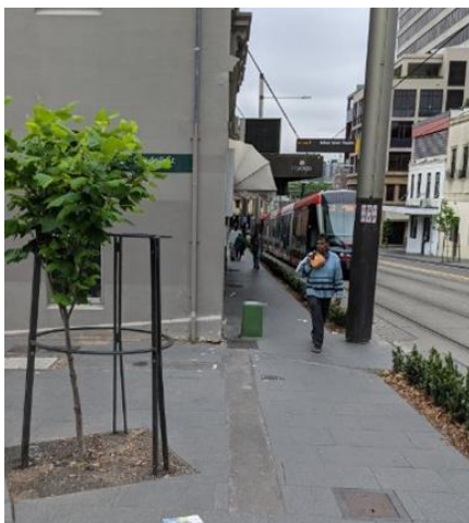
Fig B23 - Unacceptable – Low distribution pillar too close to building corner. A commercial pillar would be suitable using clearances per Table 1.
