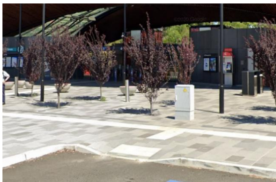
Fig B11 - Acceptable - in line with other objects, full height, marginal for 1m proximity to other fixed assets.
