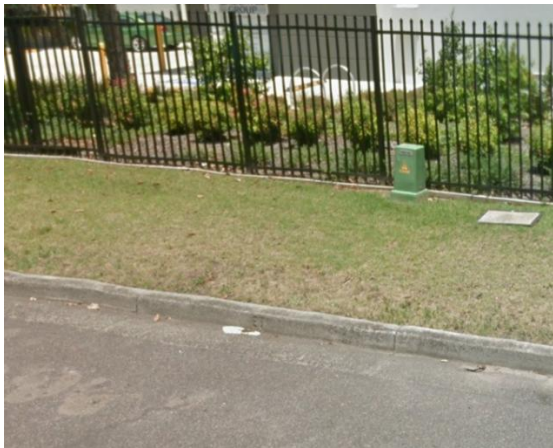
Fig B26 - Good – Clearances per Table 1 maintained, no potential trip hazard and a low impact on public safety.
