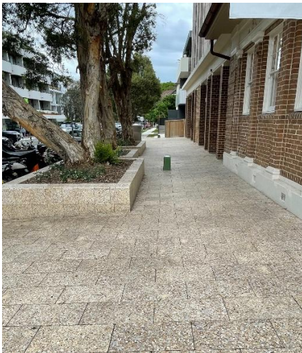
Fig B25 - Unacceptable – adjacent to property boundary, but redevelopment and new paving leaves pillar on main pedestrian thoroughfare.
