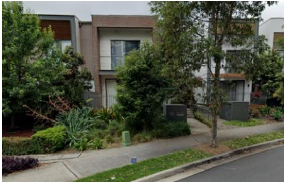
Fig B1 - Good - Clearances per Table 1 maintained. A commercial pillar is also suitable for this area.
