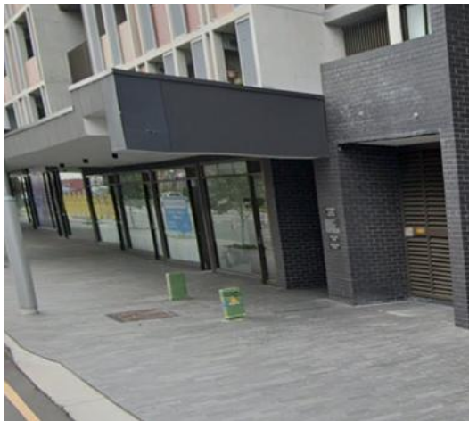
Fig B21 - Unacceptable – the pillars are adjacent to the property boundary, but the building line setback means they are in the middle of the footpath.
