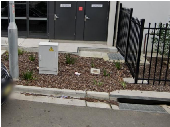
Fig B28 - Good – inside the property line and does not impede pedestrian access (future risk of garden overgrowth).
