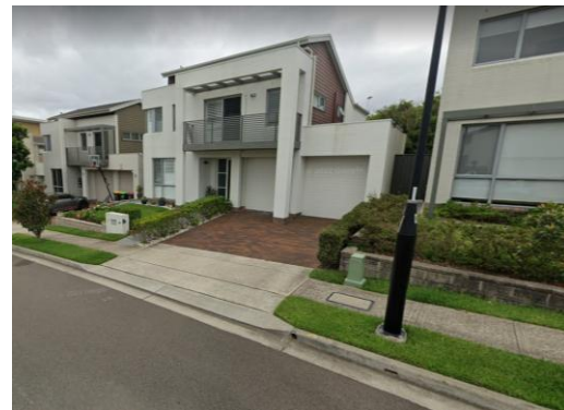
Fig B4 - Good – Clearances per Table 1 maintained
