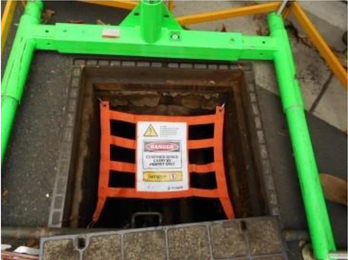
Figure 6 –Webbing sign, as installed
